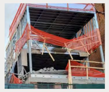
A knuckleboom deposited CMU block on a deck before the framing system was complete, overloading the deck.
